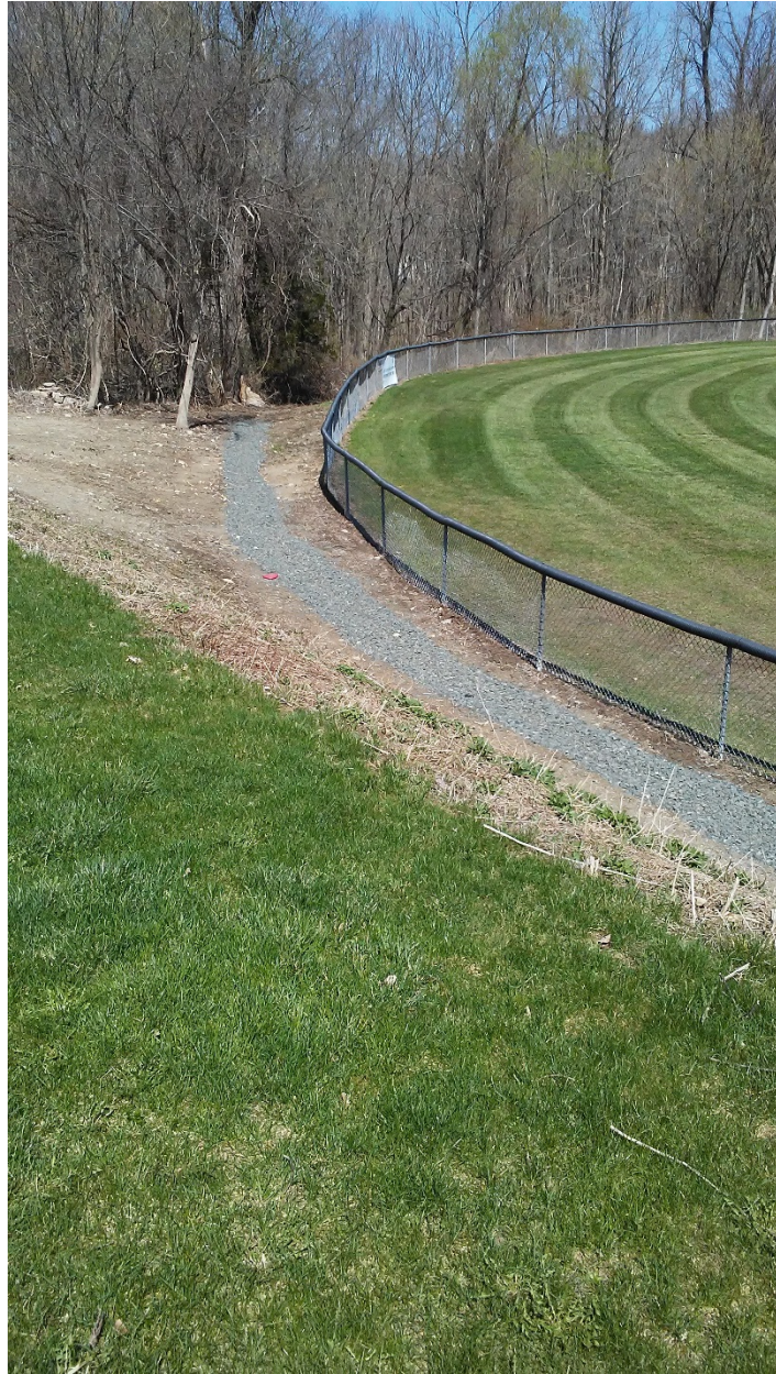
Grassed swale at toe of slope alongside baseball field
